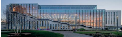
Believe in Better Building, London, UK
